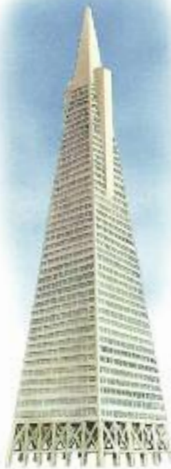
The Transamerica Building in San Francisco is specially designed to withstand even the most severe earthquakes. It is shaped like a slender pyramid and, thanks to special steel supports, its top is strong enough to sway 12 m and still remain intact. In 1989 an earthquake shook California. Its epicentre was 100 km south of San Francisco. Although quite severe, the quake damaged few buildings in San Francisco. Most had been built to resist earthquake shaking.
